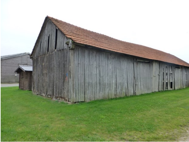
Hist. Holzscheune in Godenstedt
